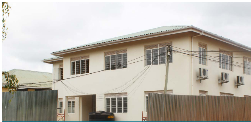
The new training building where some bioinformatics activities will be hosted.
