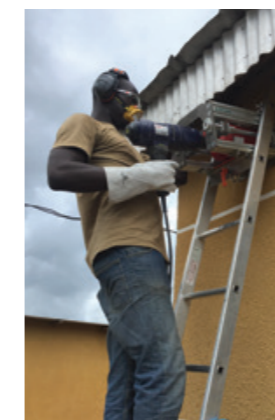
Eave tubes being installed to a house in Bouake, Cote d'Ivoire
