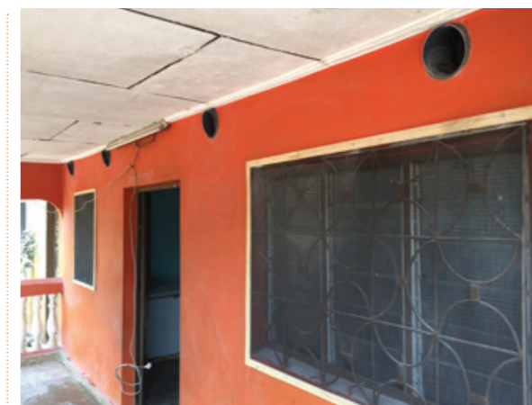
Example of a house with eave tubes and screening installed, Bouake, Cote d'Ivoire
